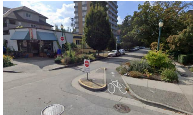
Figure 15 Example of Traffic Diversion
