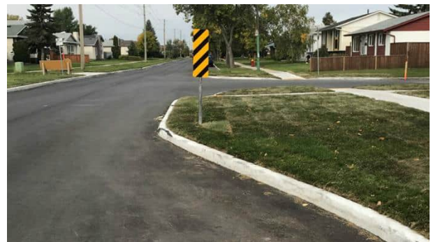
Figure 11 Curb Bump Out (City of Winnipeg)
